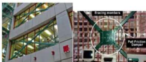
Fig.3. Pall Friction Dampers
