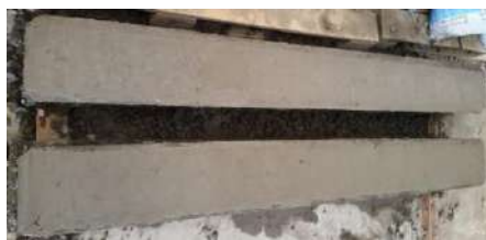
Fig. 2: Casting of Beams
