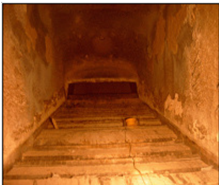
Fig. 6. Clinker phenomenon on refractory surface in furnace: (a) case of leachate, (b) case of food wastewater
