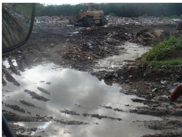
Fig. 3. A snapshot of condition of landfill and leachate in Langkawi Island (2010)
