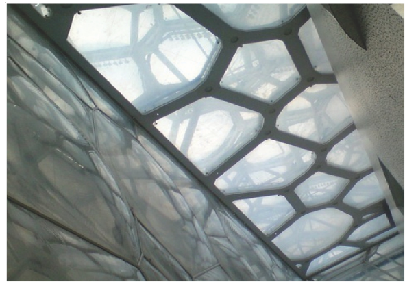
Fig. 2. Indoor natural lighting effect inside the water cube by using the ETFE membranes
