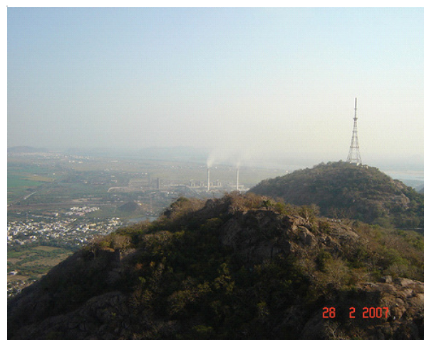
Fig. 3. Vijayawada thermal power station and environs
