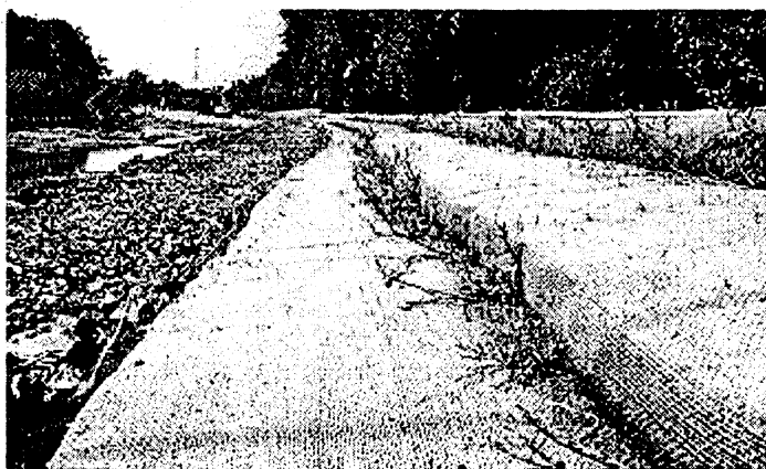
Fig. 3. An innovative coir fabric encapsulated river-bank stabilization technique
