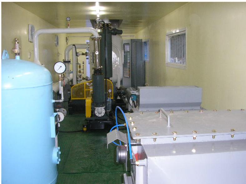
Fig. 2. Photograph of the installed soil purification system
